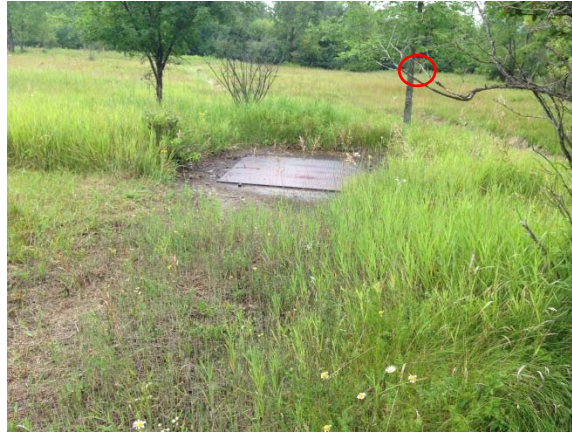
Photograph 13 - Showing rectangular concrete slab foundation with square metal cover in the vicinity of Silo no. 1 on the BU 34/35 Nike Launch Area Site. Note – Monitoring well (MW-3) located in the upper right corner (within red circle).
