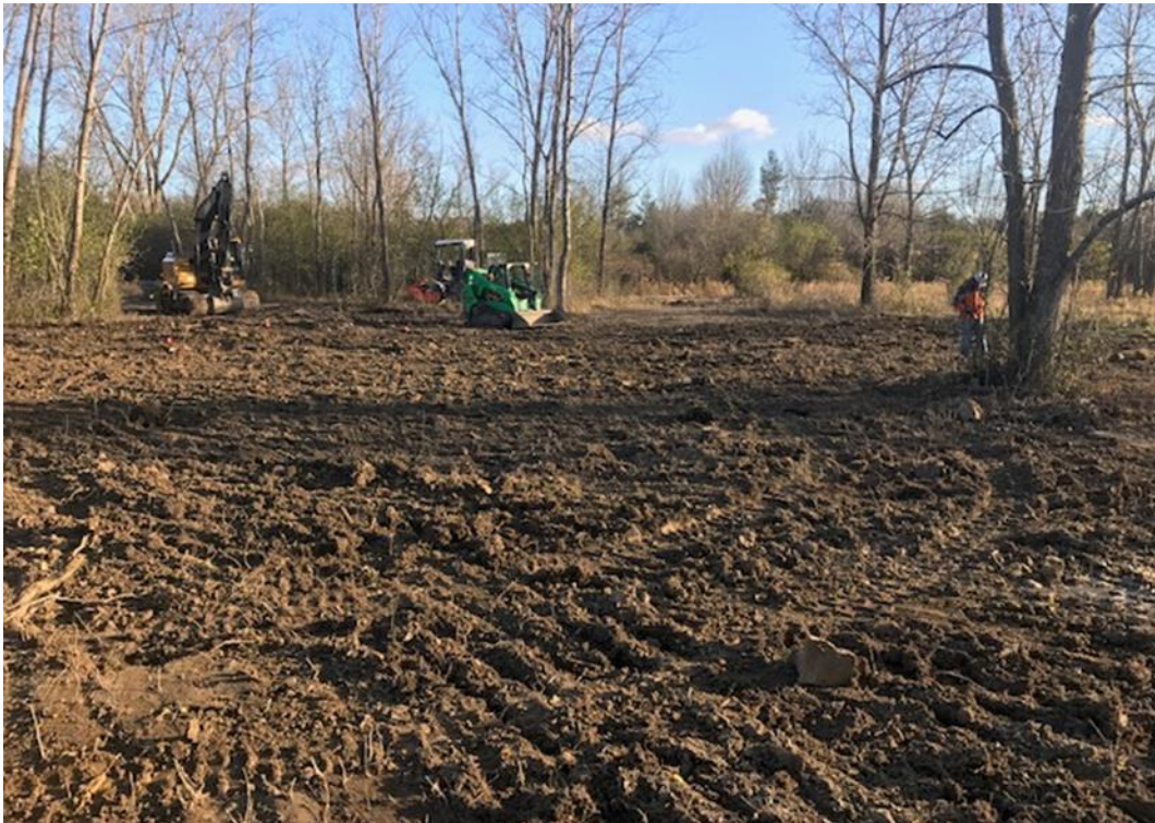
Photograph 14: Completion of backfilling (11/10/17).
