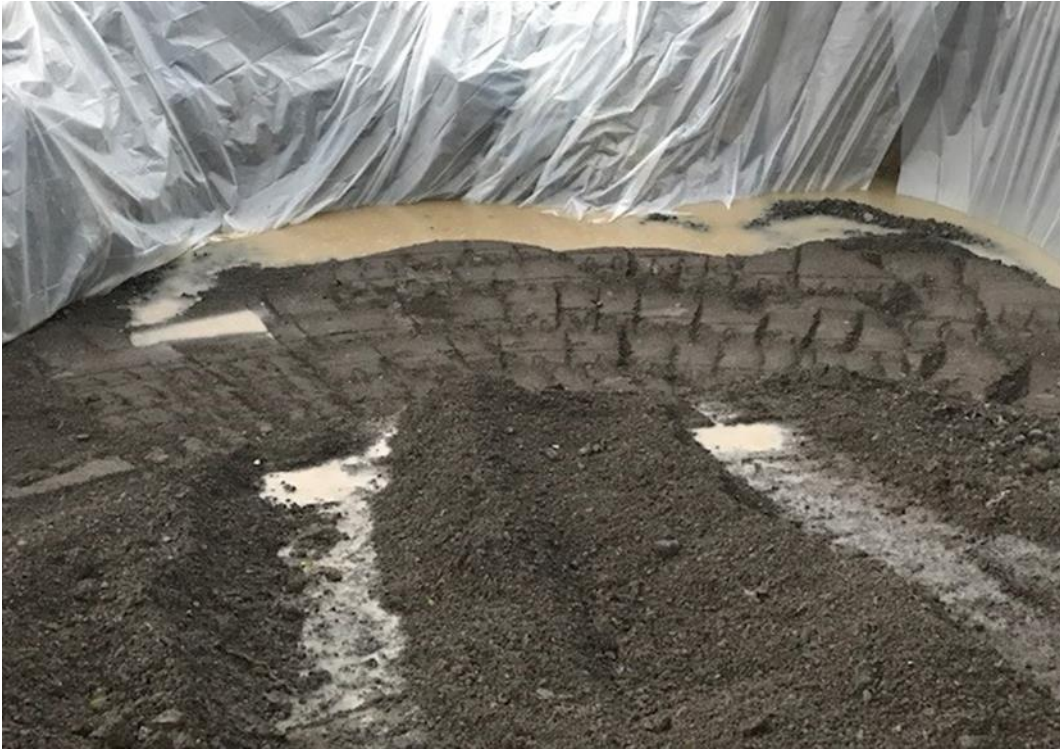
Photograph 13: Excavation being backfilled with imported gravel (11/08/17).
