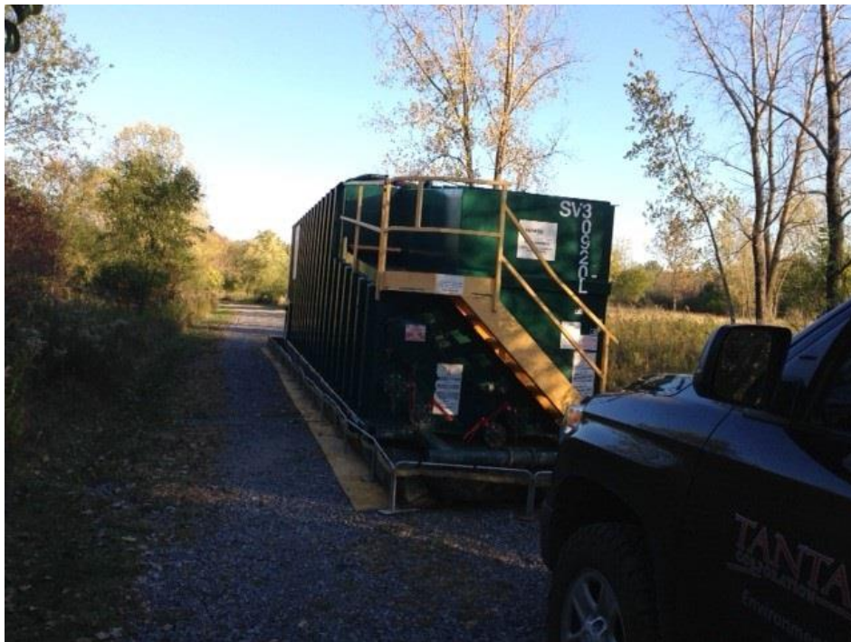
Photograph 2: Frac tank used to stage water pumped from UST and excavation (10/17/17).
