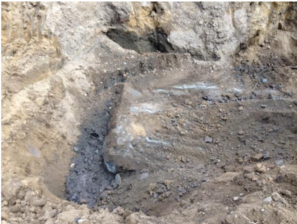
Photograph 6: Exposed west end of concrete deadman (10/25/17).
