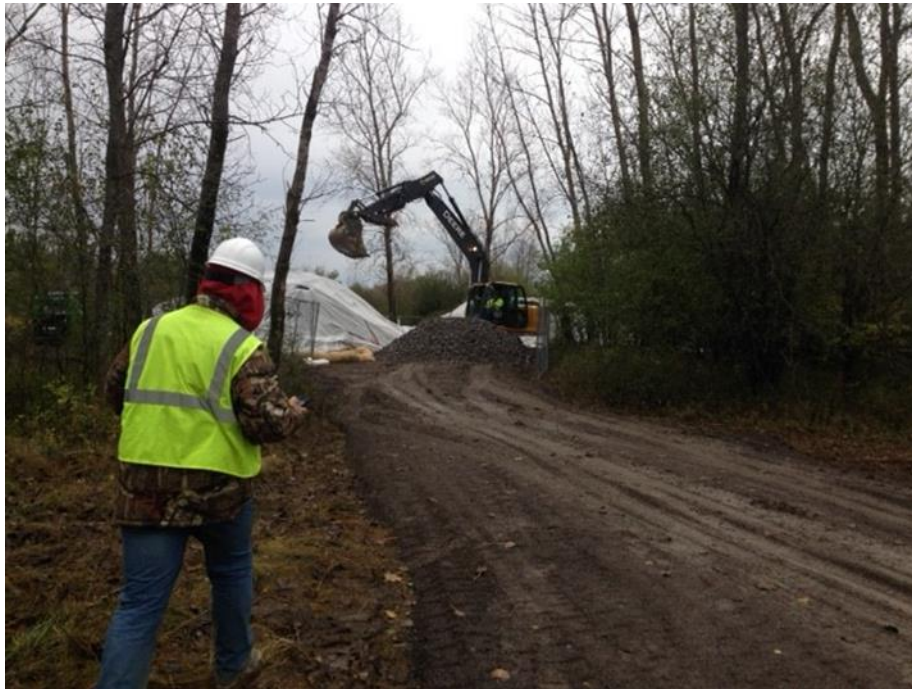
Photograph 11: Temporary gravel road installed to access soil piles for transportation to disposal facility (11/01/17).
