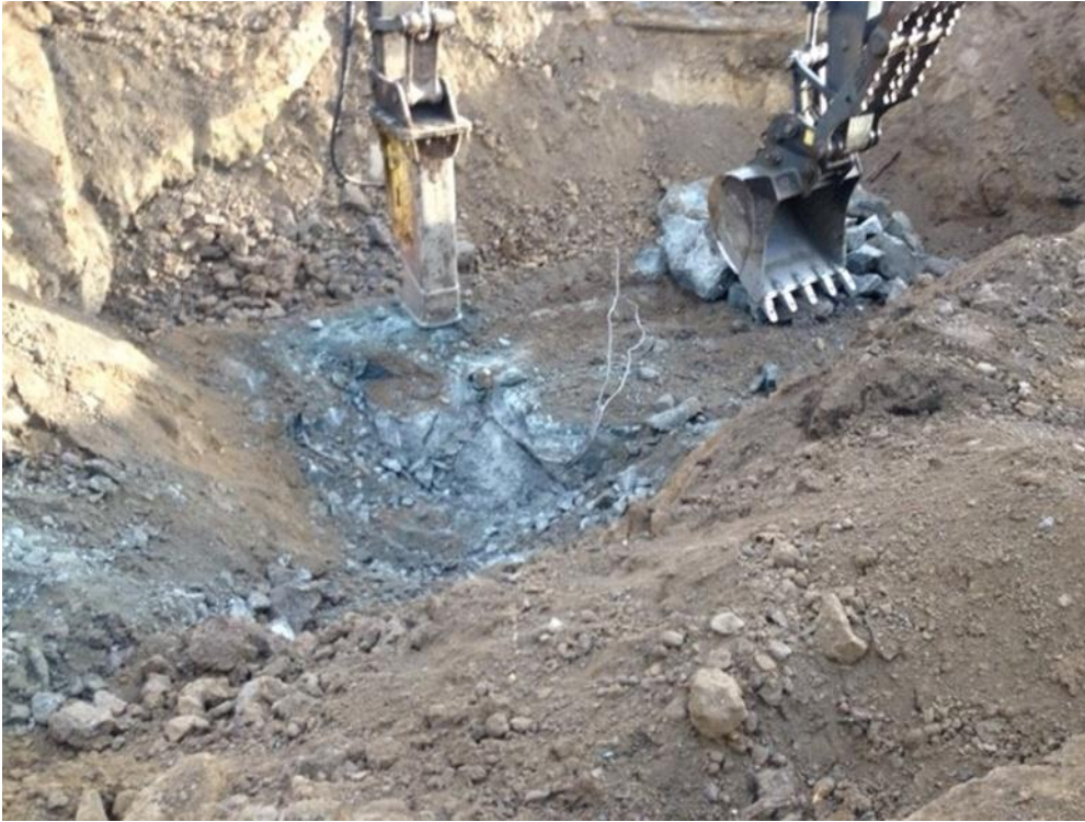
Photograph 7: Using hammer attachment to break up and remove concrete deadman (10/26/17).
