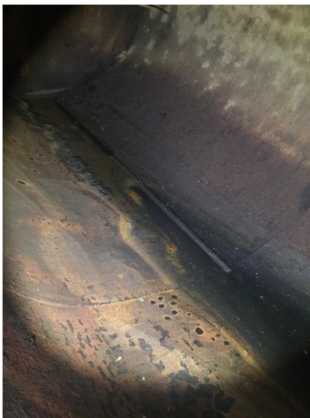
Photograph 10: Inside of UST after cleaning (10/31/17).
