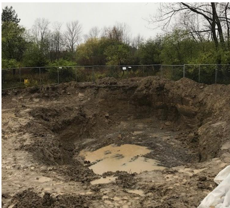
Photograph 9: Final limits of excavation prior to backfilling (10/31/17).
