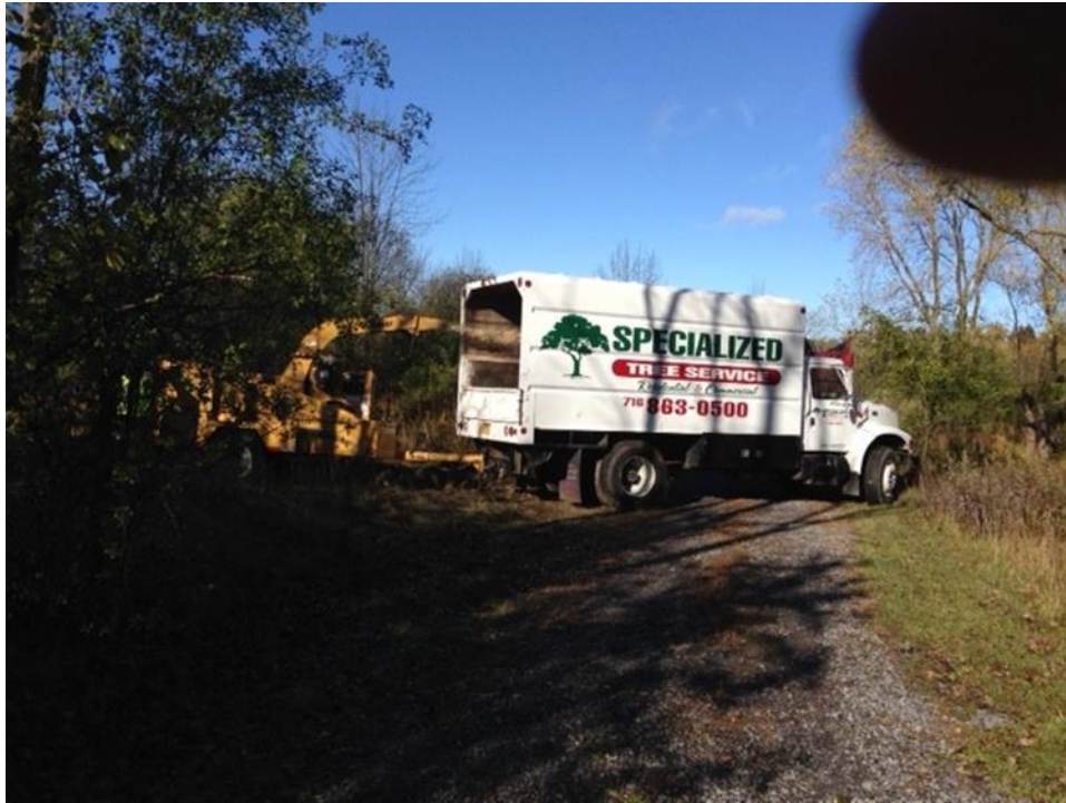
Photograph 3: Specialized Tree Service chipping trees removed from around excavation (10/24/17).
