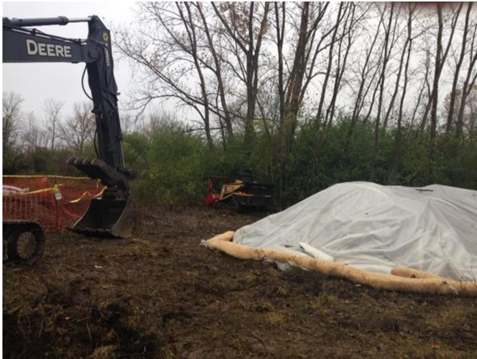
Photograph 5: Soil stockpile covered with poly sheeting (10/25/17).
