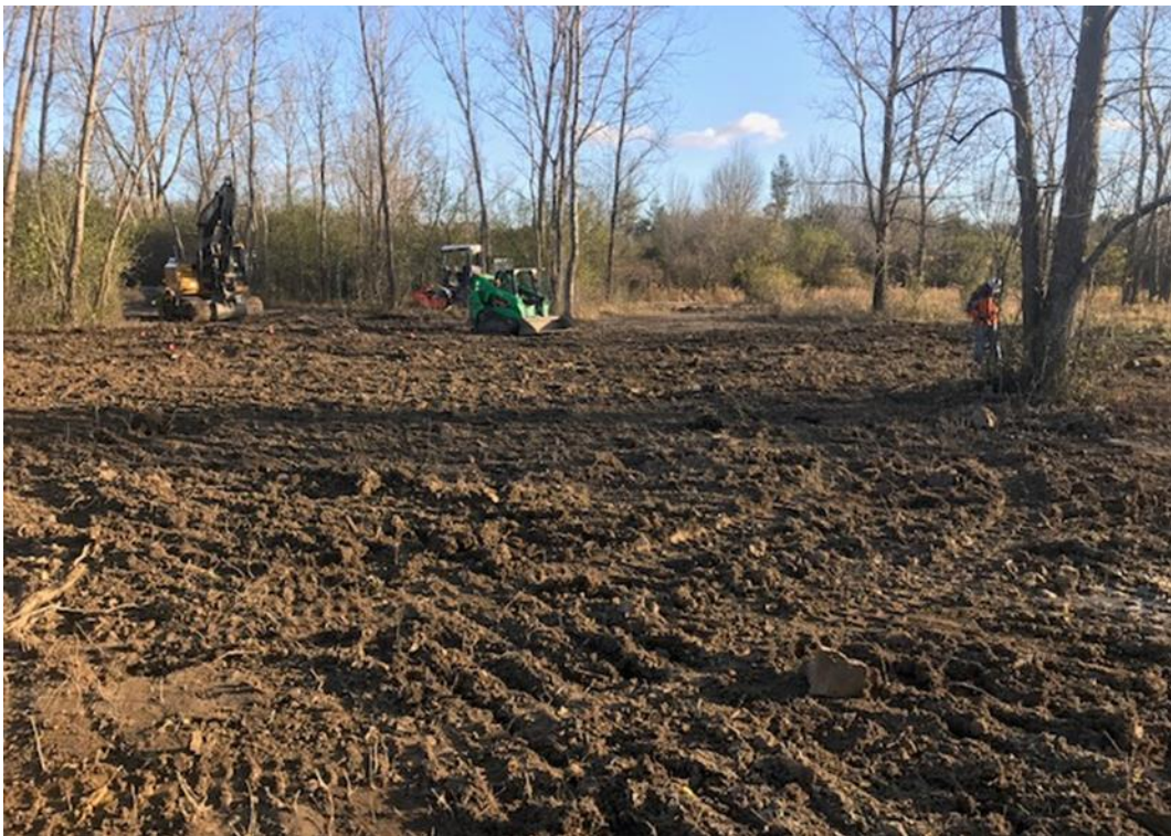
Photograph 14: Completion of backfilling (11/10/17).
