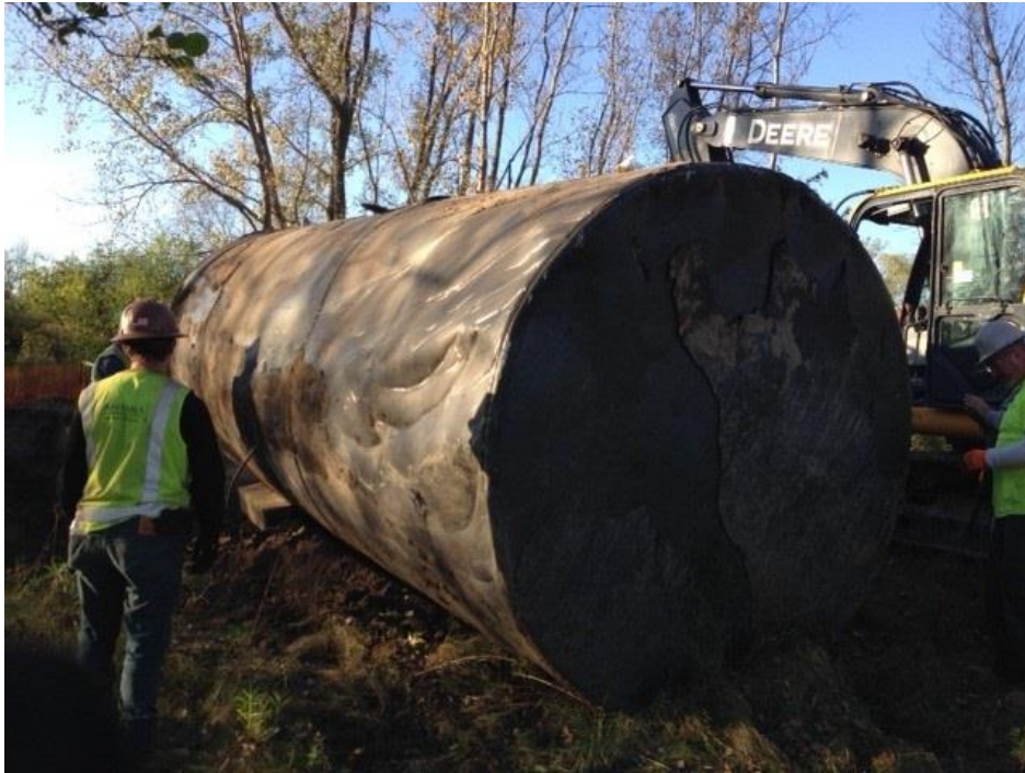
Photograph 1: UST after removal from excavation (10/17/17).
