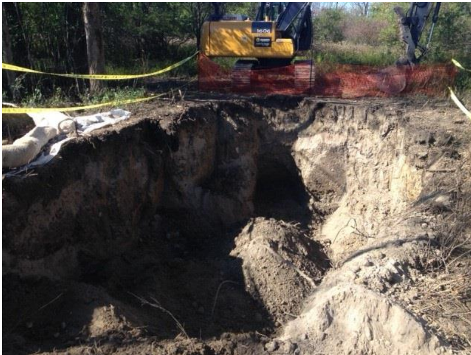
Photograph 4: Extent of excavation on 10/18/17.
