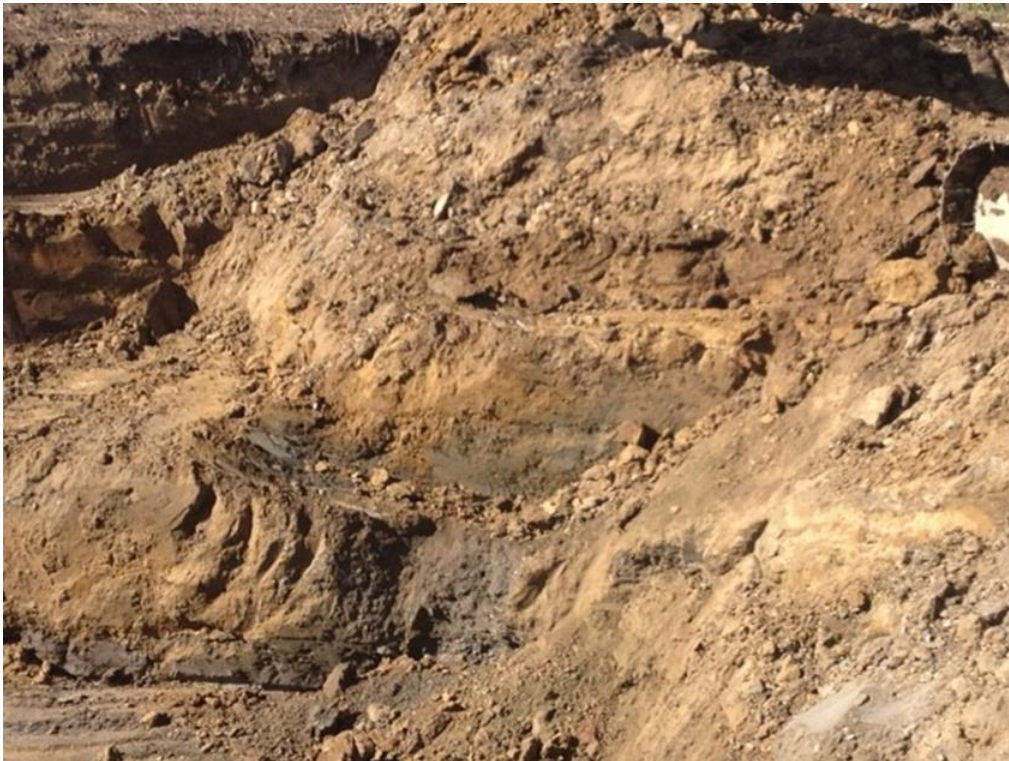
Photograph 8: West side of excavation. Gray colored soil determined to be native clay (10/26/17).
