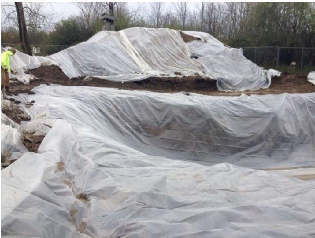
Photograph 12: Excavation lined with poly sheeting prior to backfilling (11/01/17).
