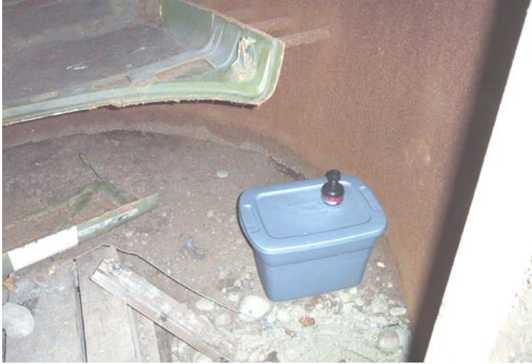
Tank Interior 2 – A second radon electret is visible on the plastic bin. The other hood and wood pallet are on the left.
