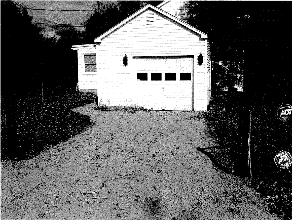
Photo 57 – Site Restored – Ms. Burns Driveway
