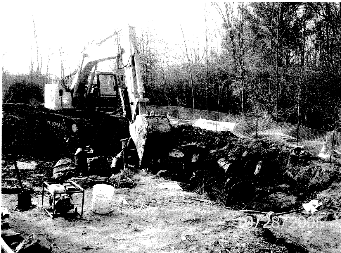
Photo 14- Area D Excavation
