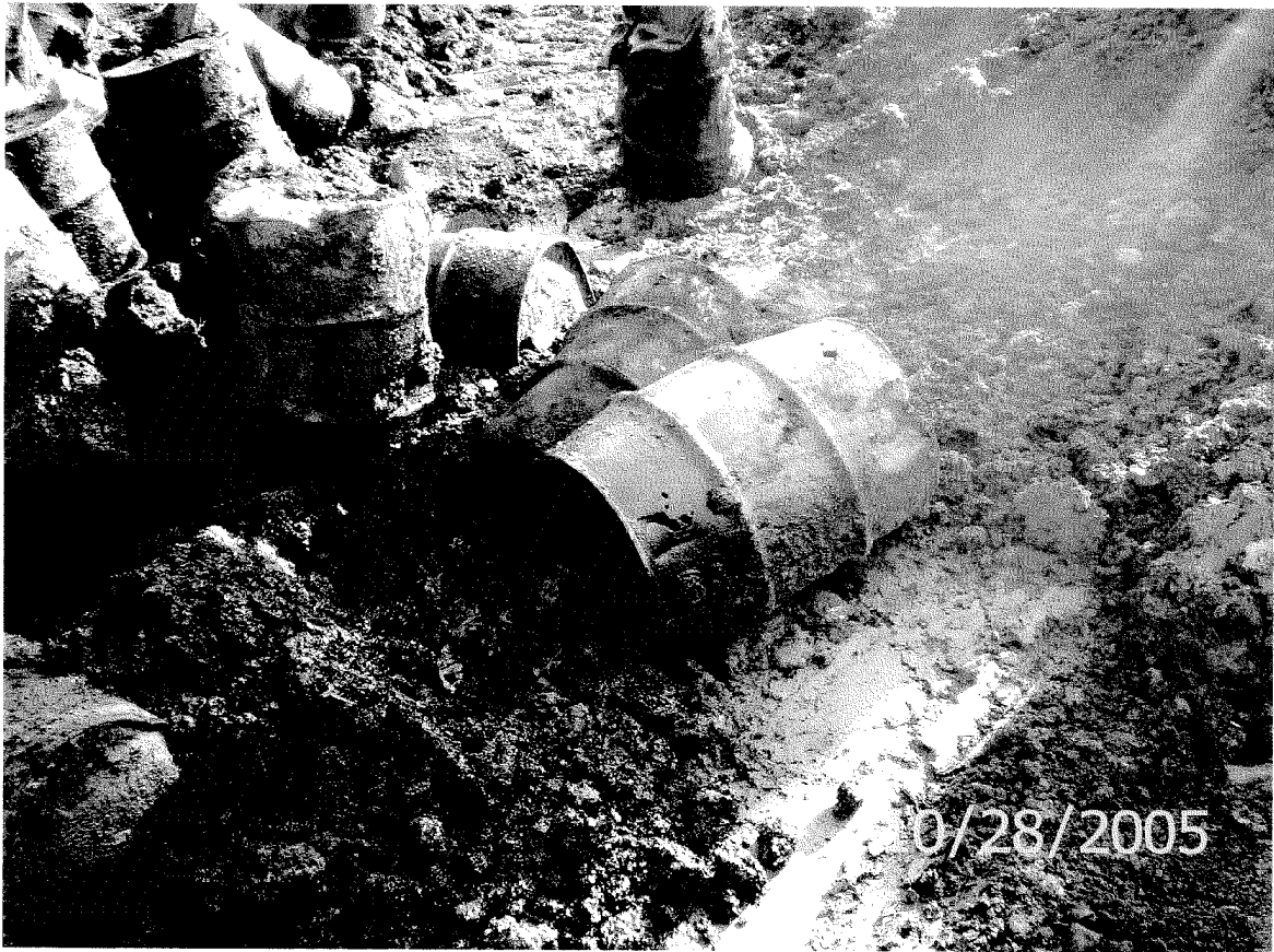
Photo 13 - Area D Excavation
