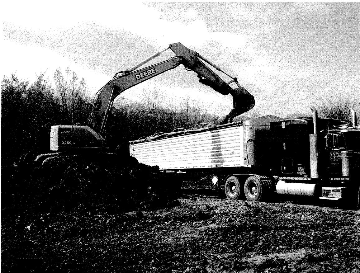
Photo 45– Soil Load Out (2006)
