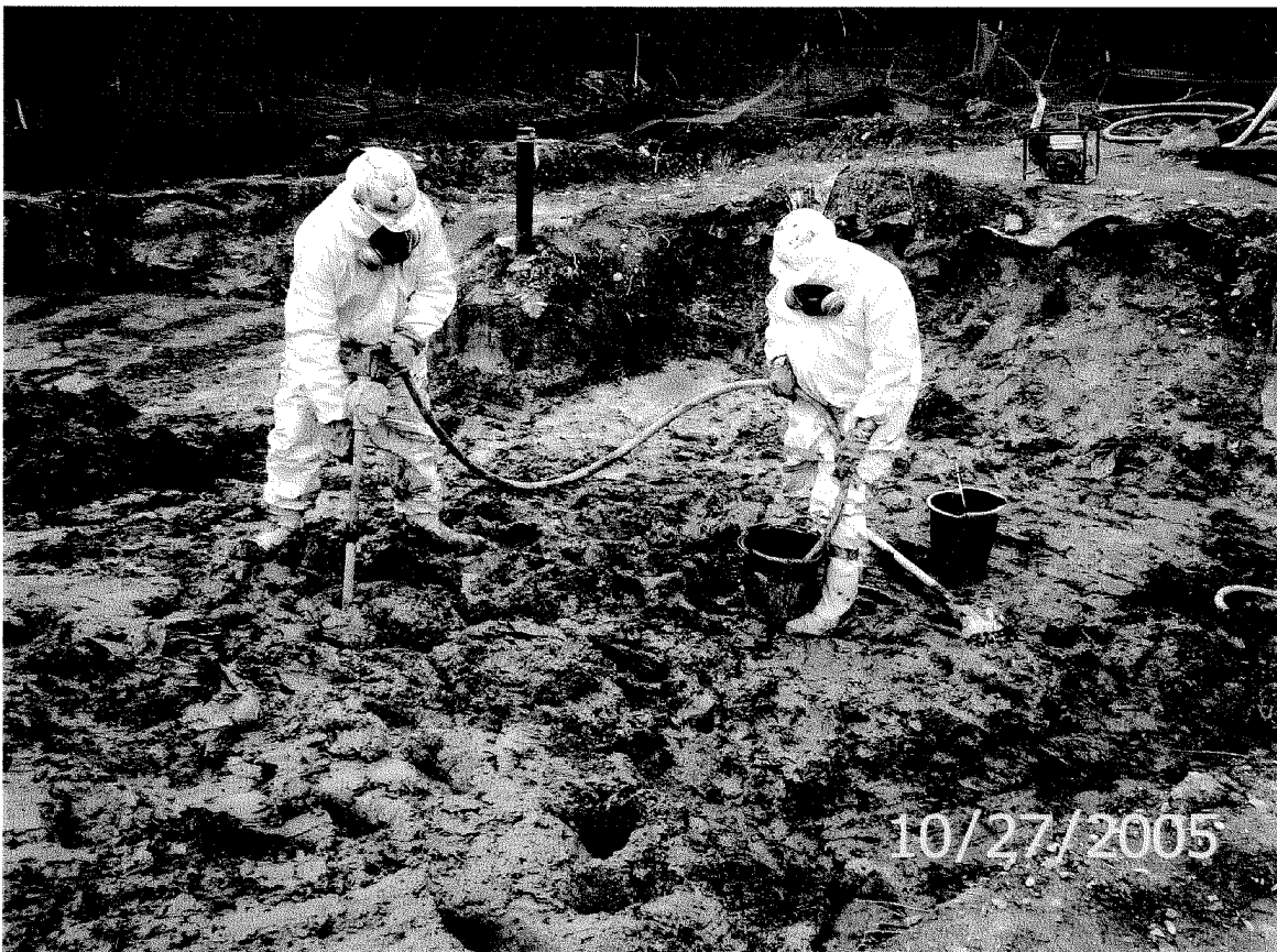
Photo 10 – Area D – Drum Product Removal
