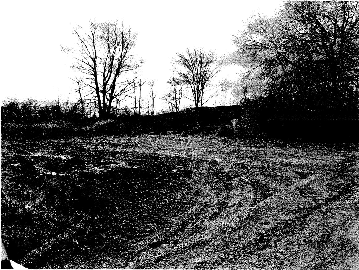
Photo 55 – Site Restored – Office Trailer Area
