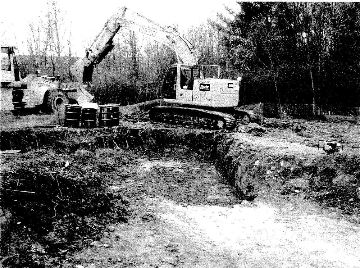
Photo 4 – Area D Excavation (2005)
