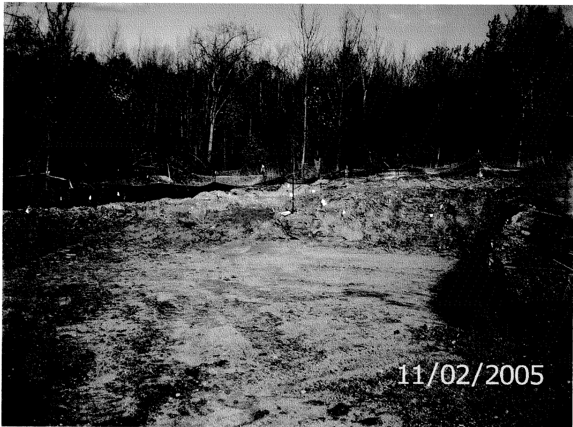
Photo 8- Area B/C Excavation
