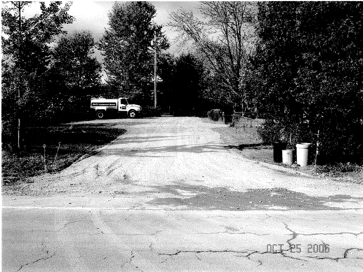
Photo 60 – Site Restored – Ms. Burns Driveway
