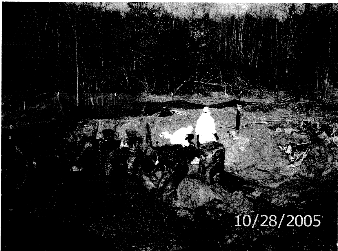
Photo 12- Area D Excavation
