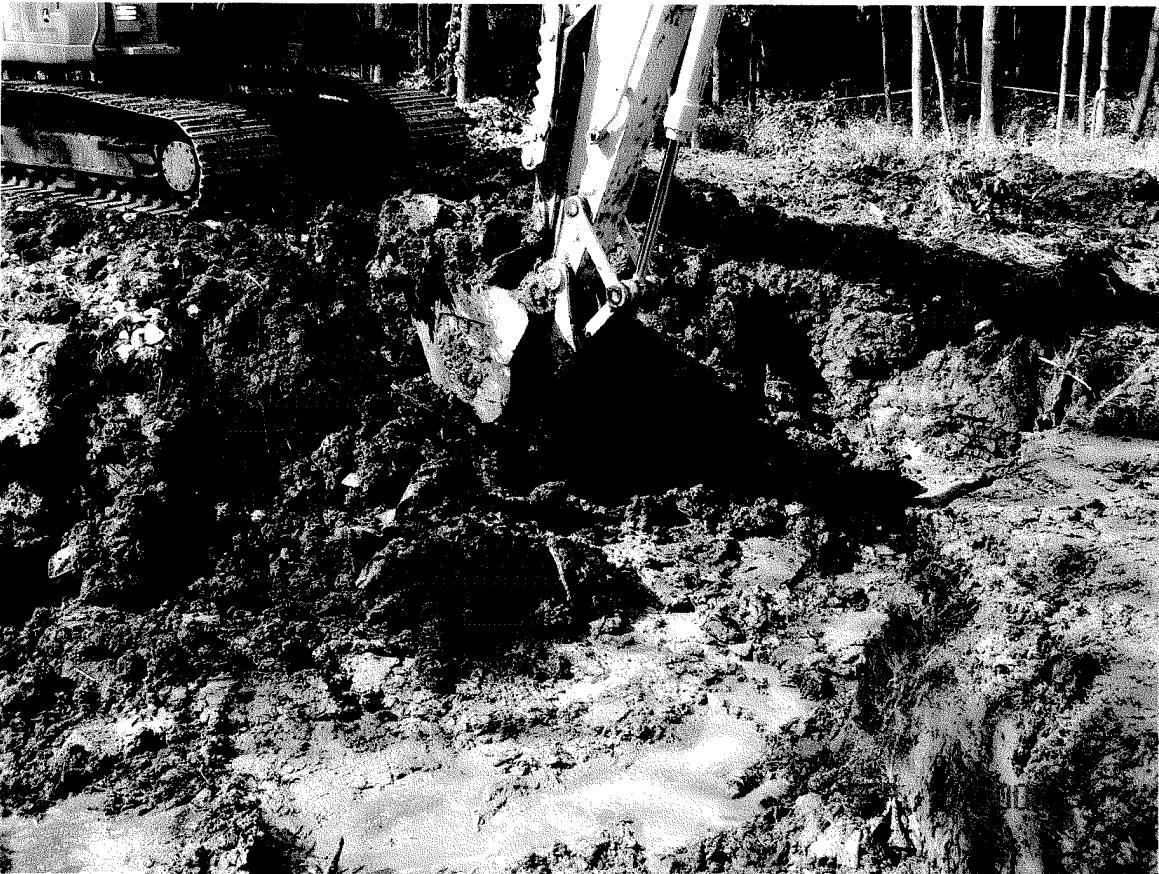
Photo 26– Area F Excavation – Continuing (Drum Carcasses)
