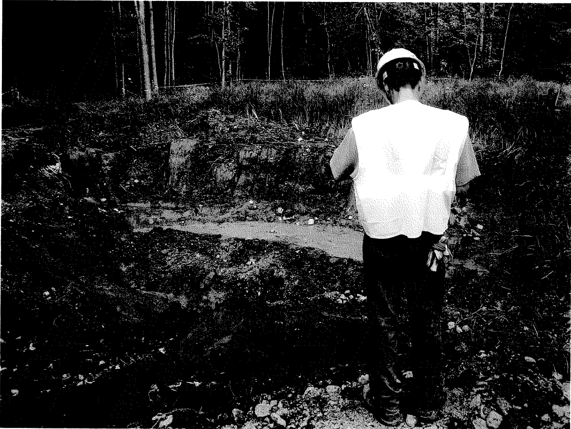
Photo 28 – Area F Excavation
