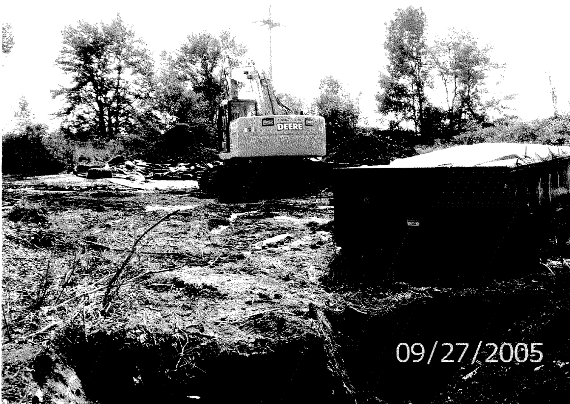
Photo 20 – Soil Load-out Operation (2005)
