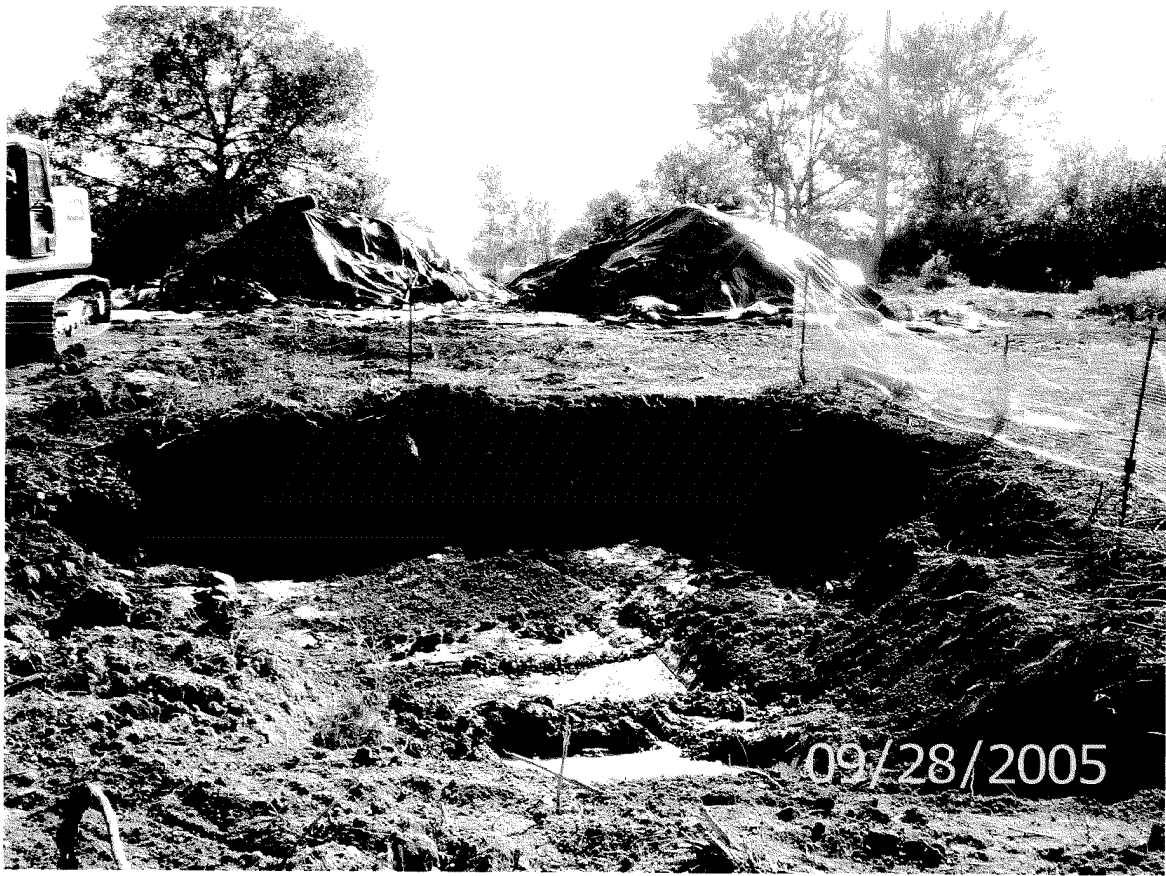
Photo 7 - Area B/C Excavation
