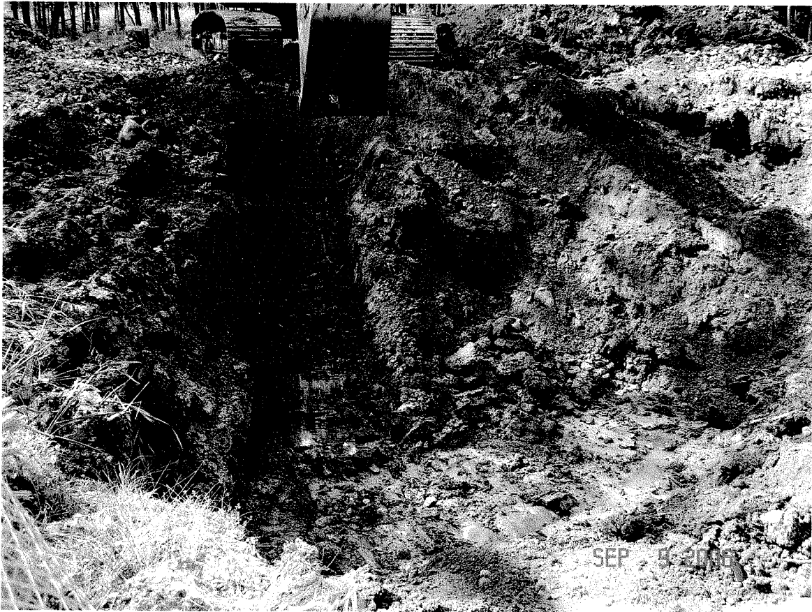
Photo 27- Area F Excavation – Slit Trench Extending South to 'Clean Fill'
