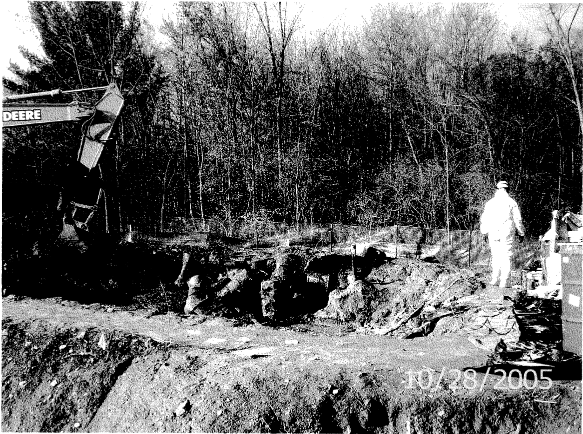
Photo 11- Area D Excavation
