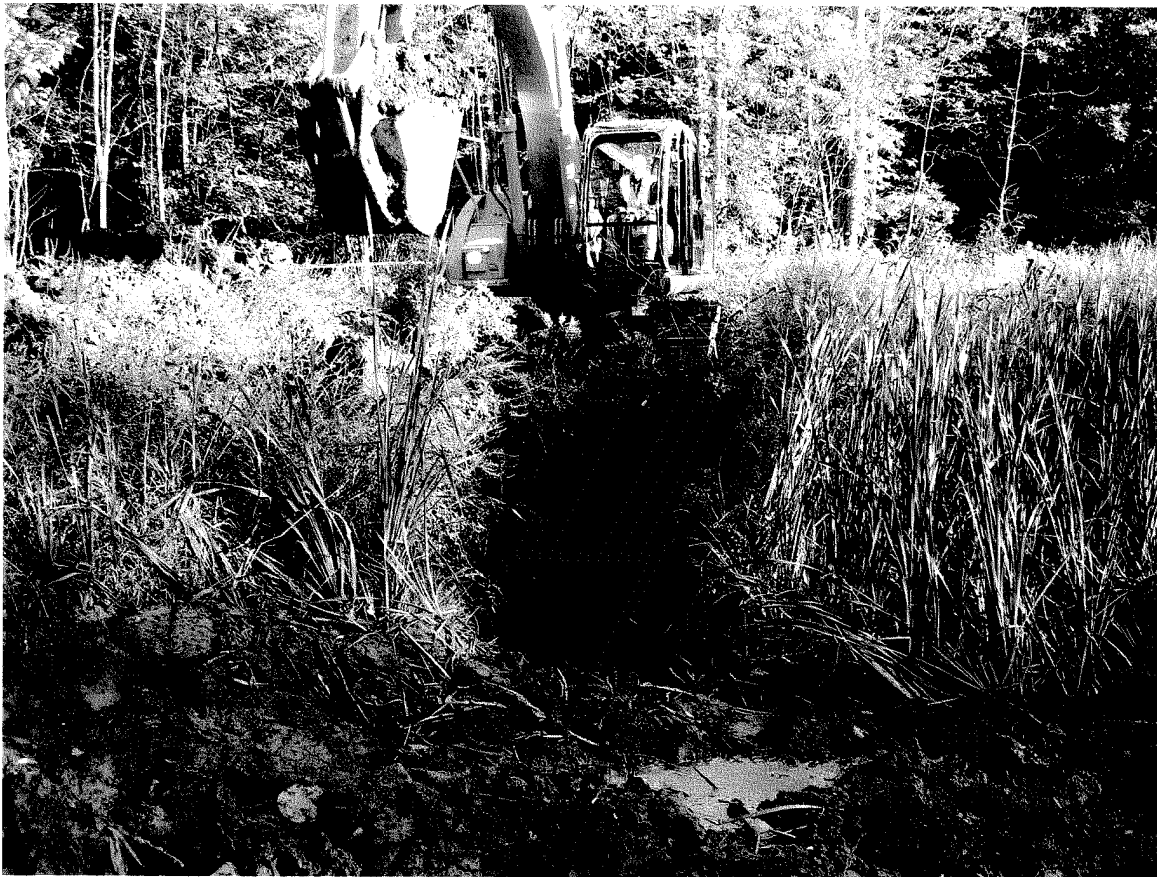
Photo 29 - Area F Excavation – Slit Trench North of Area F (2006)
