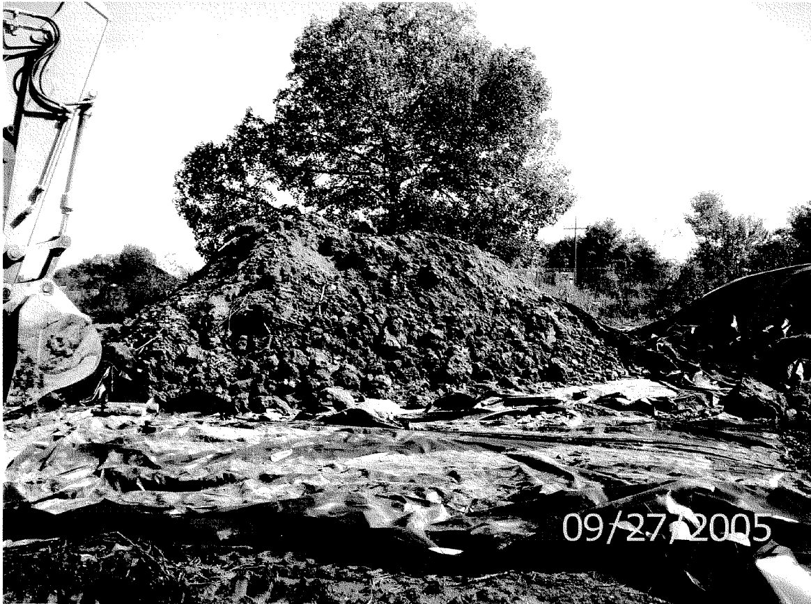
Photo 19- Soil Load-out Operation (2005)
