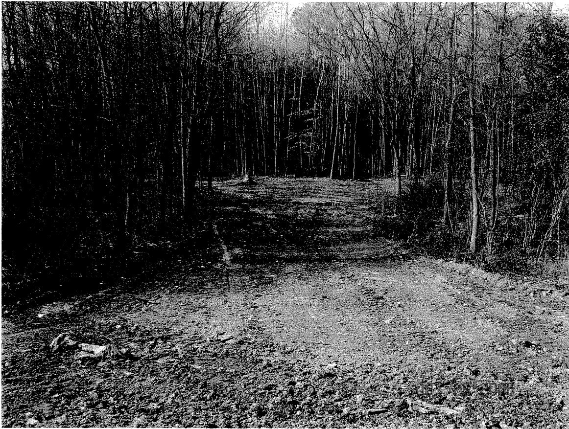
Photo 47 – Site Restored – Main Haul Road West to Area F
