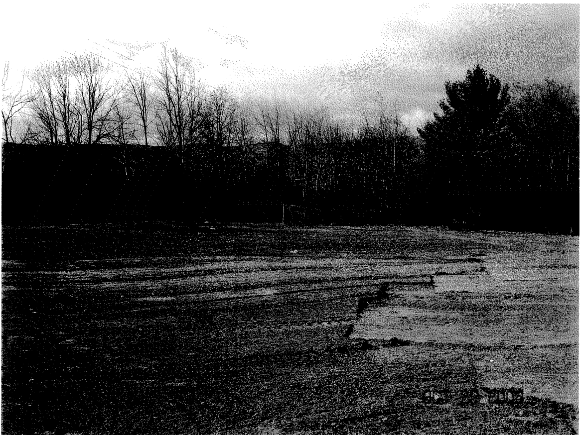
Photo 54– Site Restored – Soil Staging Area
