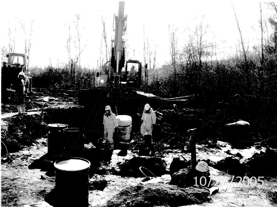
Photo 15 - Area D Excavation
