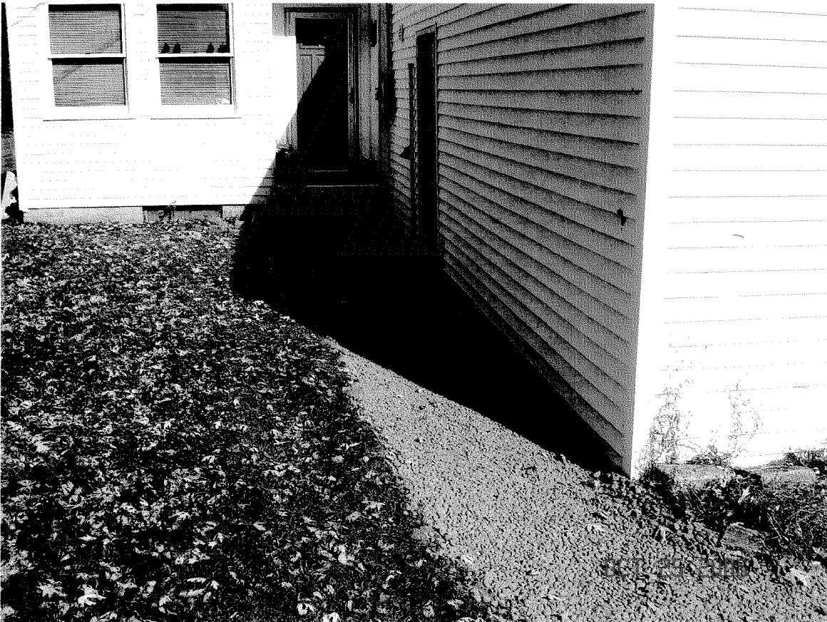
Photo 58– Site Restored – Ms. Burns Sidewalk
