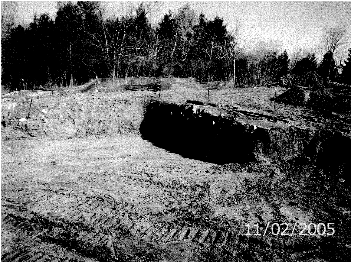
Photo 9- Area B Excavation
