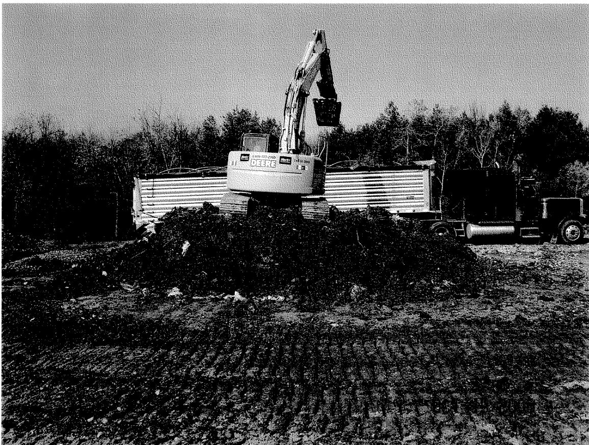
Photo 46 – Soil Load Out (2006)
