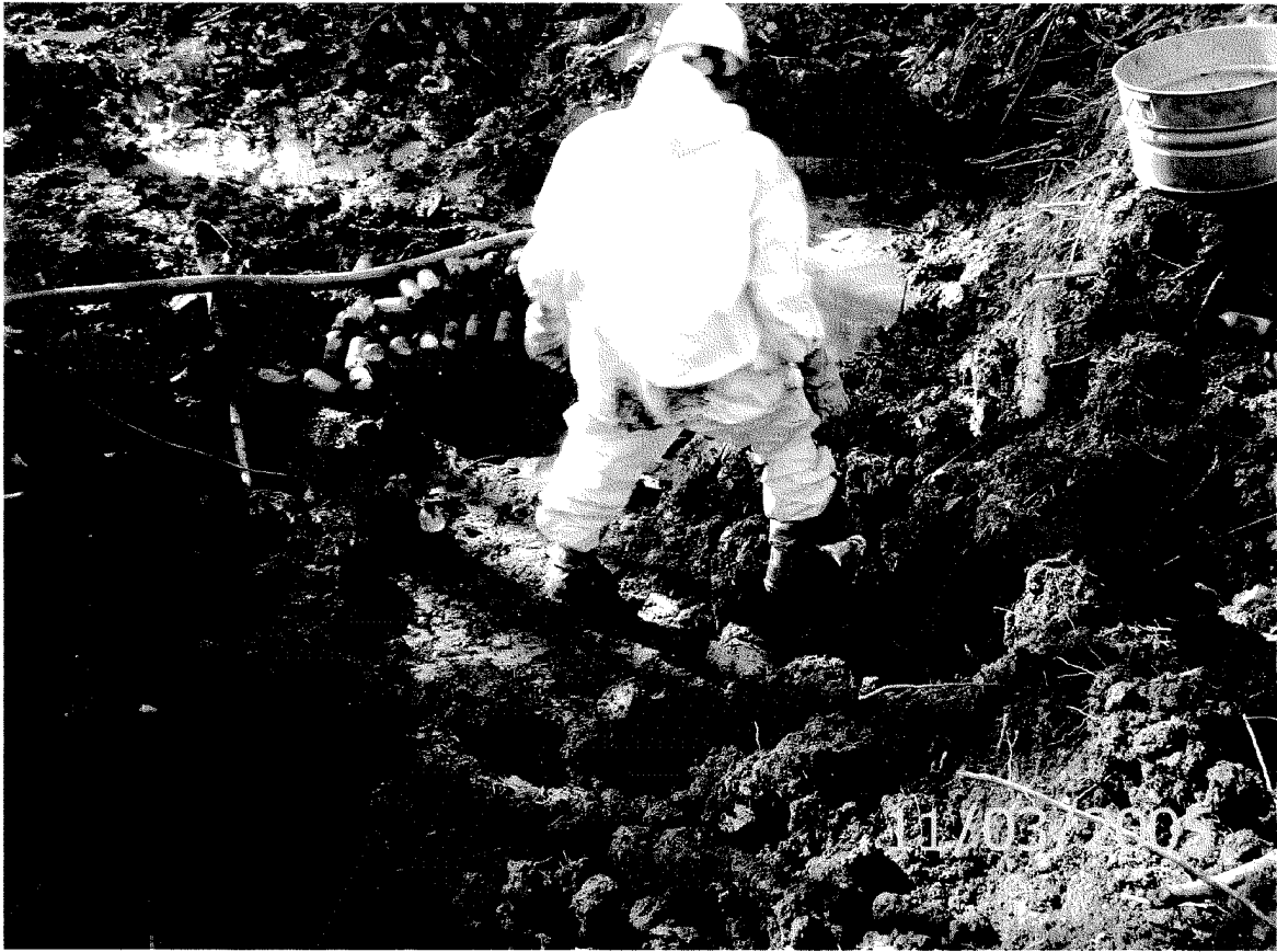
Photo 5 - Area F Excavation (2005)
