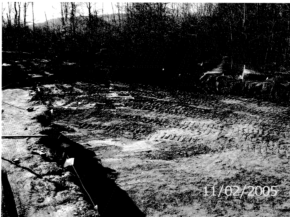
Photo 16 - Area D Excavation
