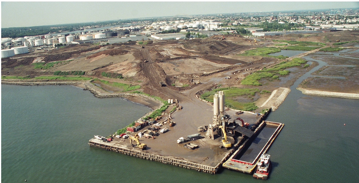
Dredged material being used to cap a brownfield in Bayonne, New Jersey, circa 2000
