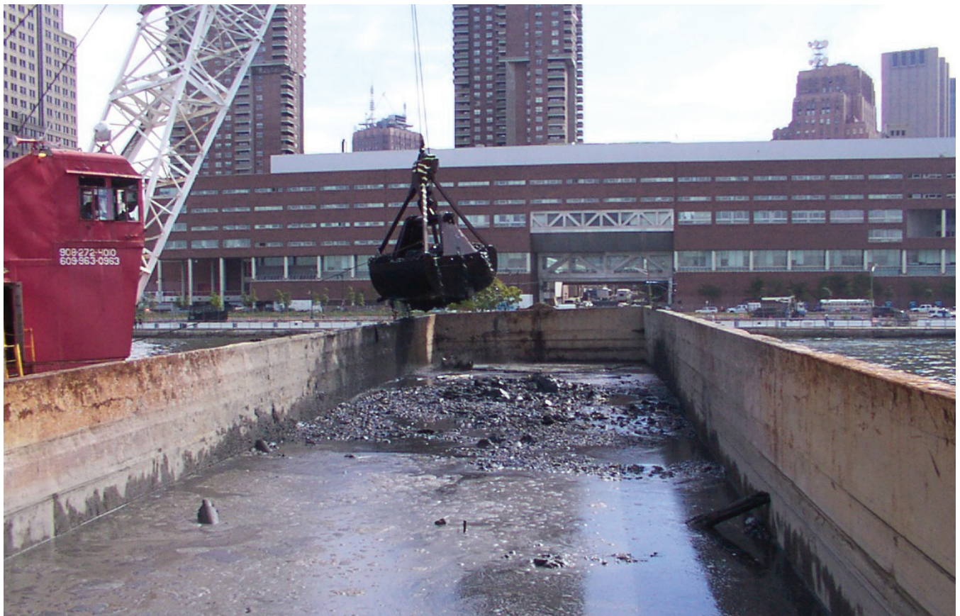
Clamshell dredge at work at Pier 25
