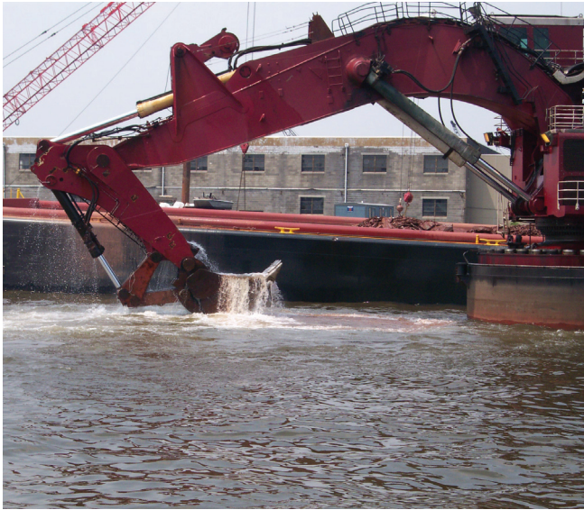
A dredge at work loading a barge in the New York-New Jersey harbor, circa 2000
