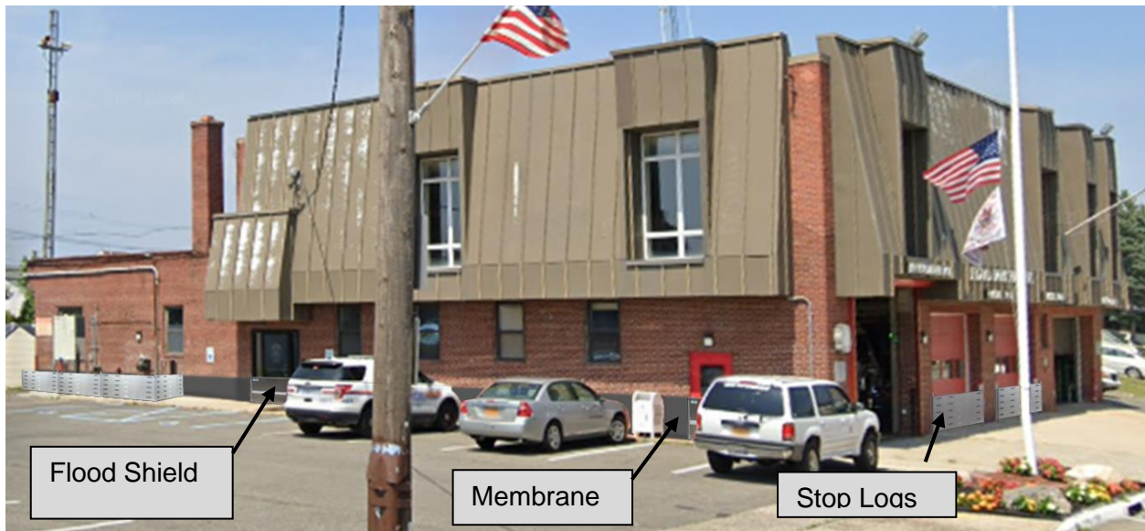
Figure 4: Street View Example of Dry Flood Proofing
